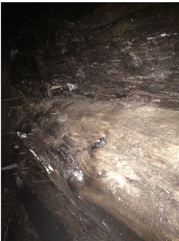
Typical stringer condition
