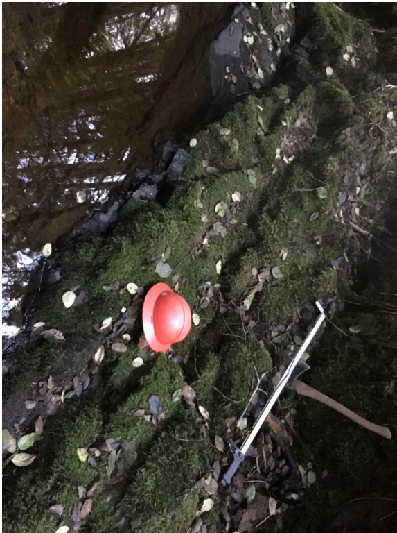
Channel bedrock, 5m upstream of bridge.
